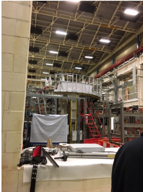
MAST upgrade from a distance
